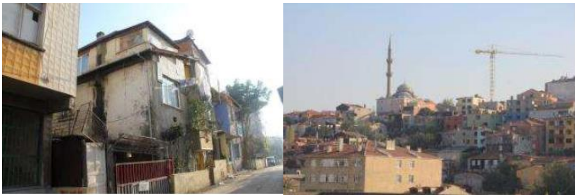
Figure 7. A view of the buildings in Fikirtepe that do not have architectural integrity and are suspicious for engineering services.
